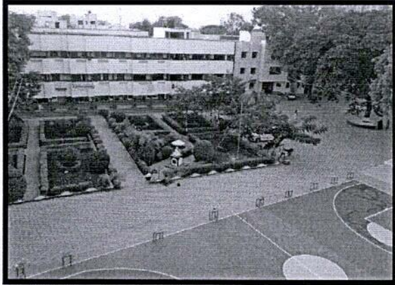
WING-I ADMINISTRATIVE BUILDING
